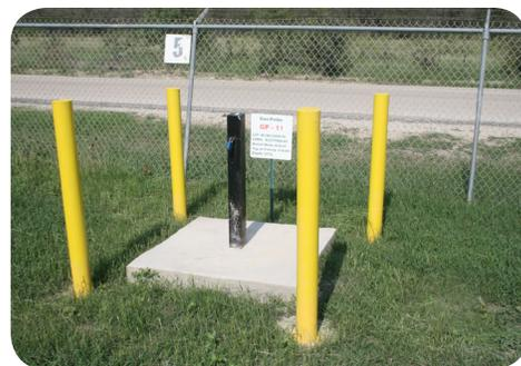
Gas probes, like the one above, are installed around the landfill. They are tested on a regular basis to determine if landfill gas is migrating off the site.
