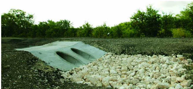
Drainage improvements are designed to manage storm water run-off and control erosion.
